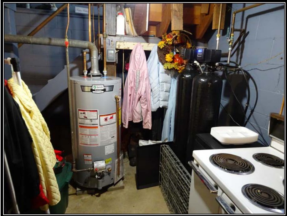
Newer hot water heater and water softener
